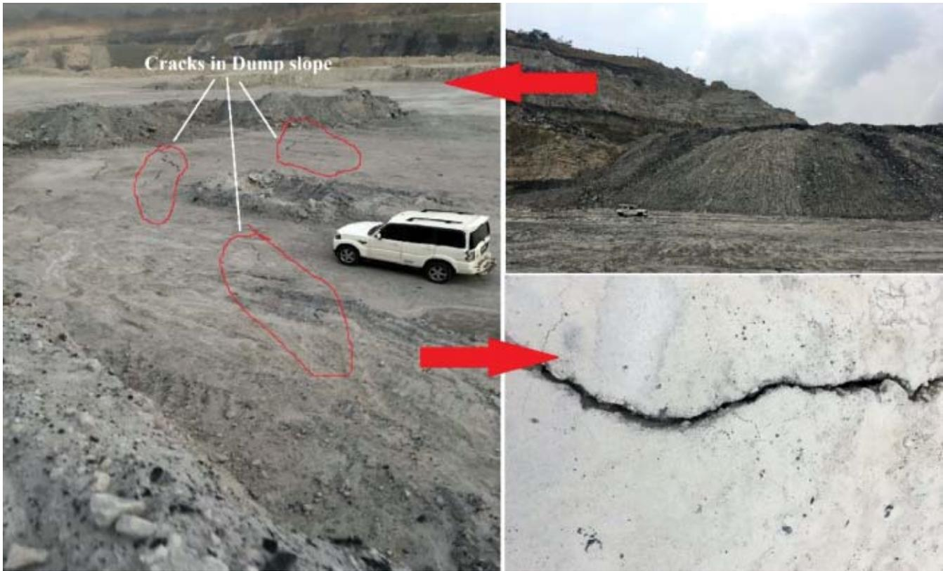
Fig.1 Cracks in the dump slope of an opencast mine
