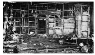
7. Fire at AMRI Hospital in Kolkata on December 9, 2011 caused death of 89 and left 67 injured. Cause was attributed to using the basement of the seven-floor structure as a storehouse with combustible substances like beds and switching-off of the fire alarm system, which resulted in the choking to death of the victims on the upper-floors.
